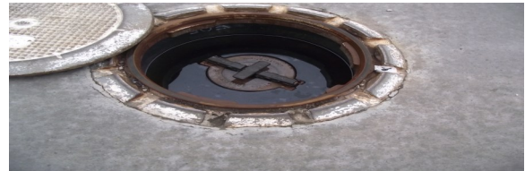
Flooded spill bucket with water entering UST through loose fill riser cap
